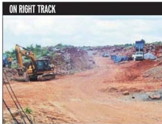
Work in progress on Southern Peripheral Road.
